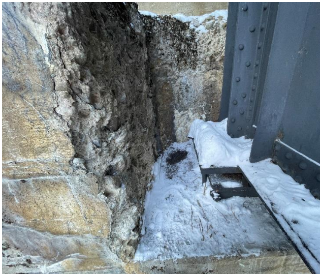
Figure 2-5: Right abutment back wall at downstream bearing.
