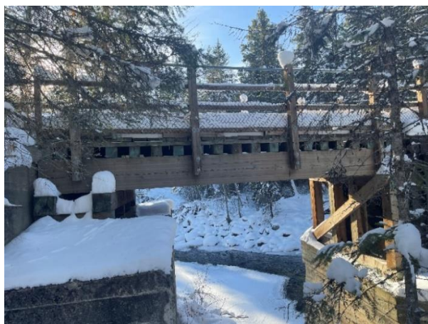
Figure 2-1: Timber approach span.
