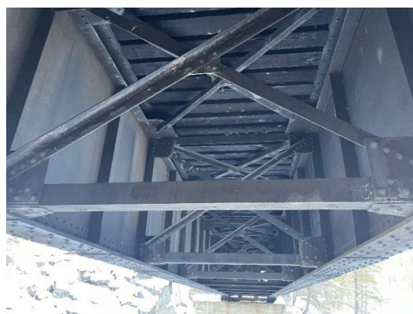
Figure 2-2: Steel girder main span.
