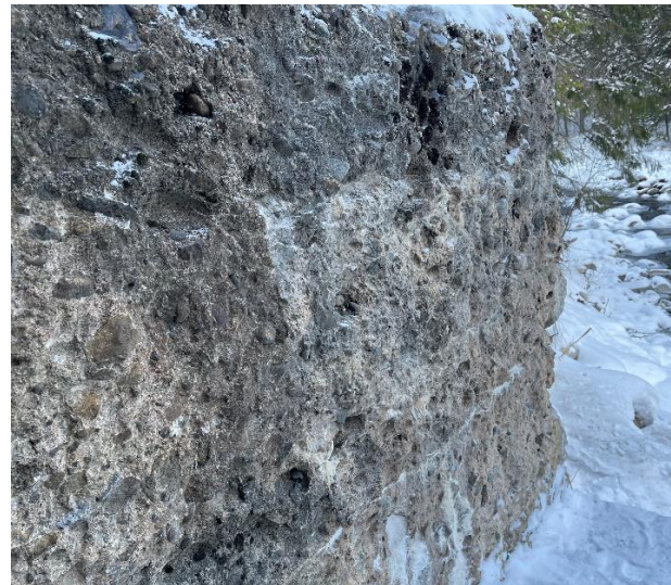
Figure 2-6: Right abutment back wall (looking upstream).
